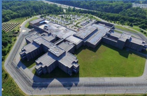
Image: Montgomery County Maryland Correctional Facility Powered by a Campus Microgrid
