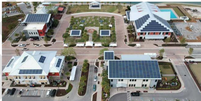
Figure 8. Babcock Ranch Solar Micro Community North of Ft. Myers, Florida
